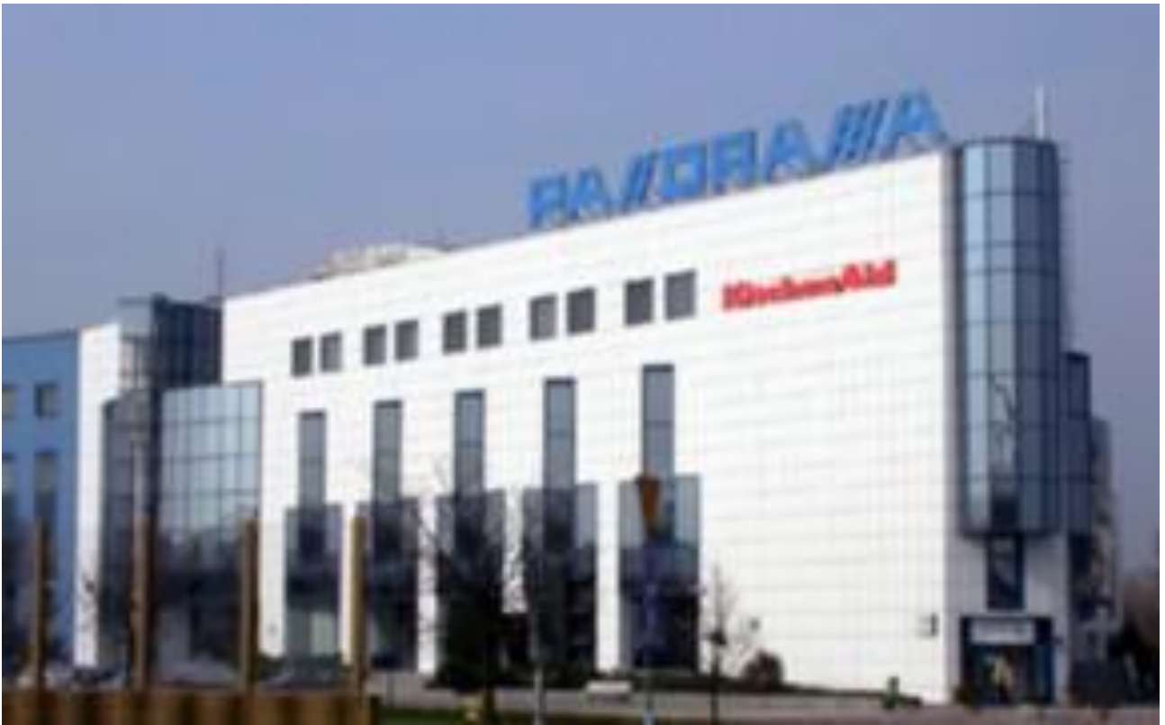
Panorama Commercial Center – Warsaw, Poland
