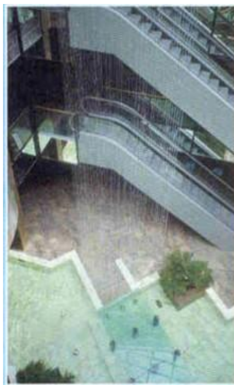
Panorama Commercial Center – Warsaw, Poland
