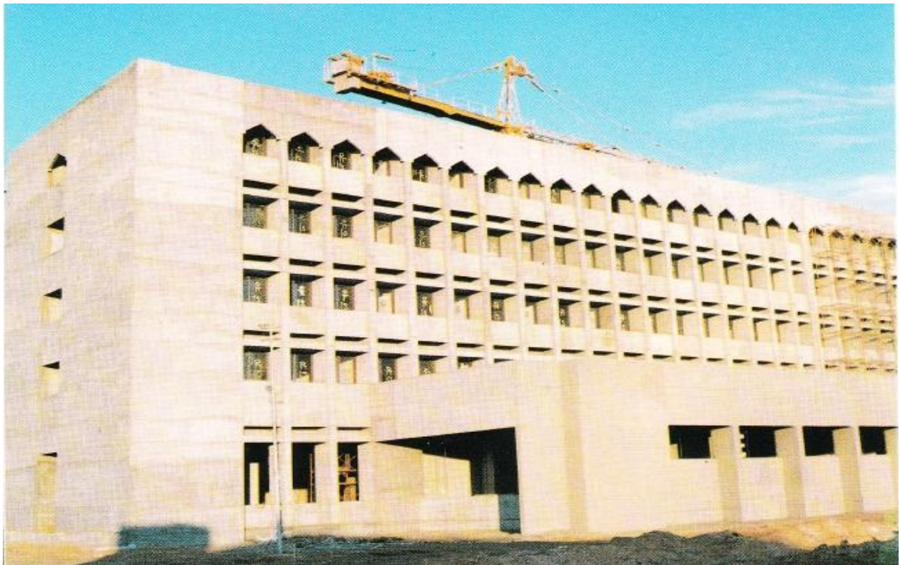
AGOCO Head Quarters – Benghazi, Libya
